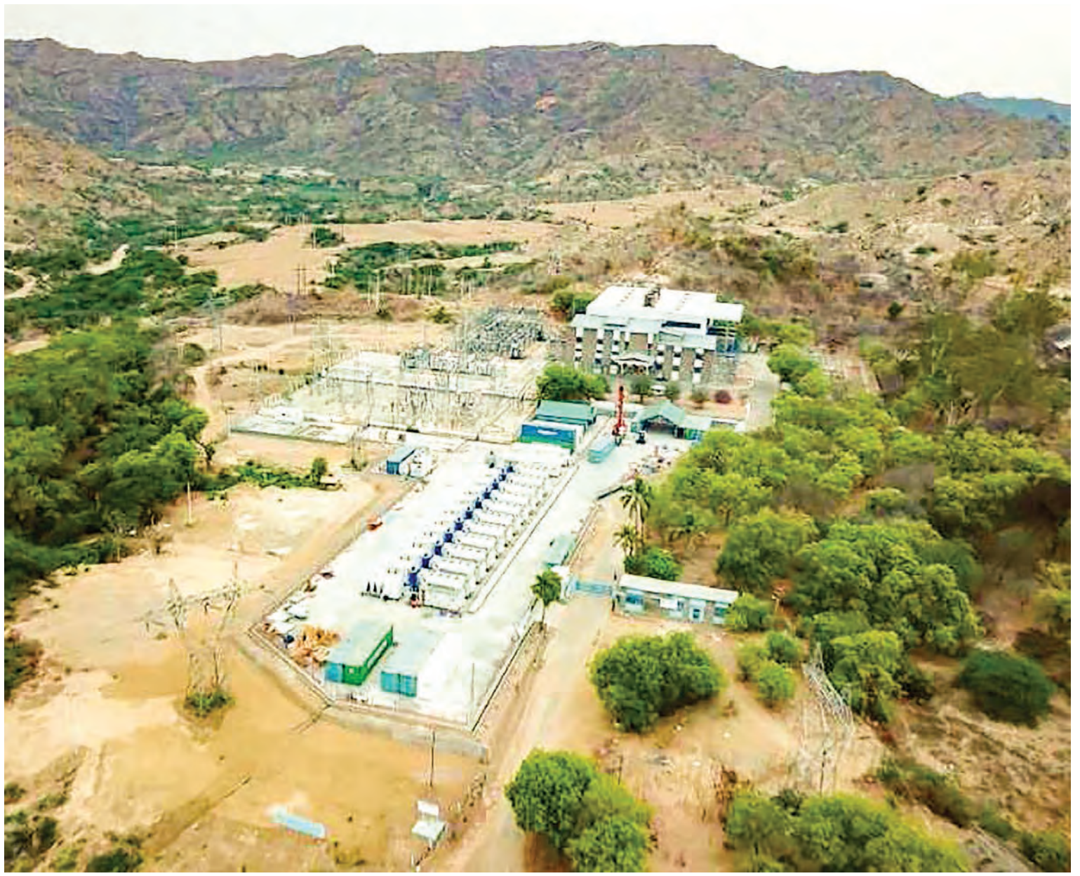
Kyun Chaung power plant.
